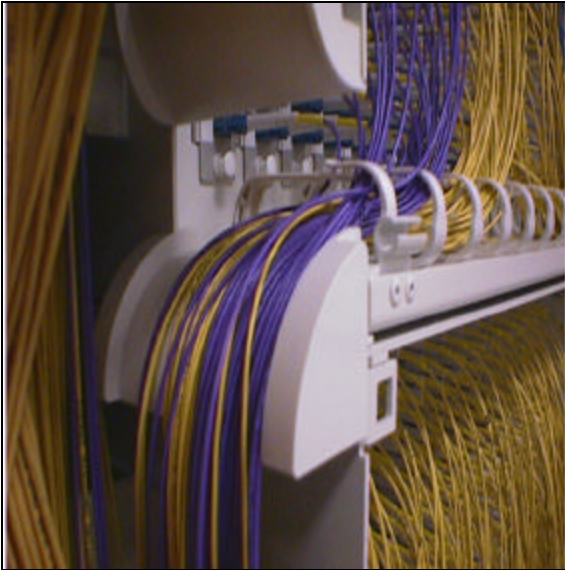
Fiber Distribution Shelf with LC 1.6-mm jumper
