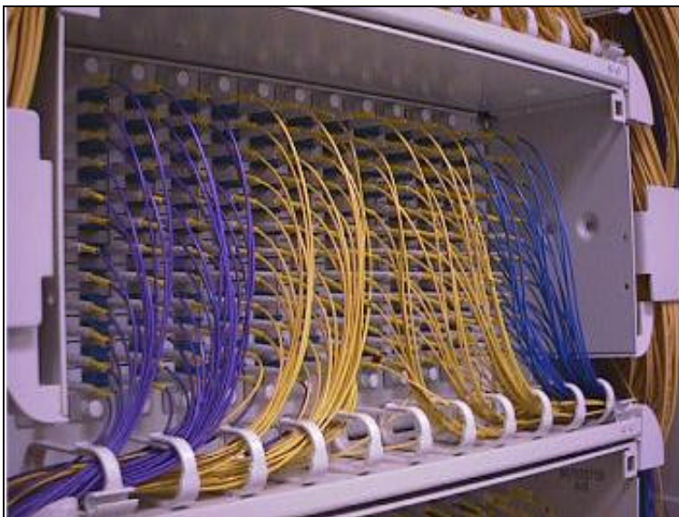
Fiber Distribution Shelf with LC 1.6-mm jumpers.
