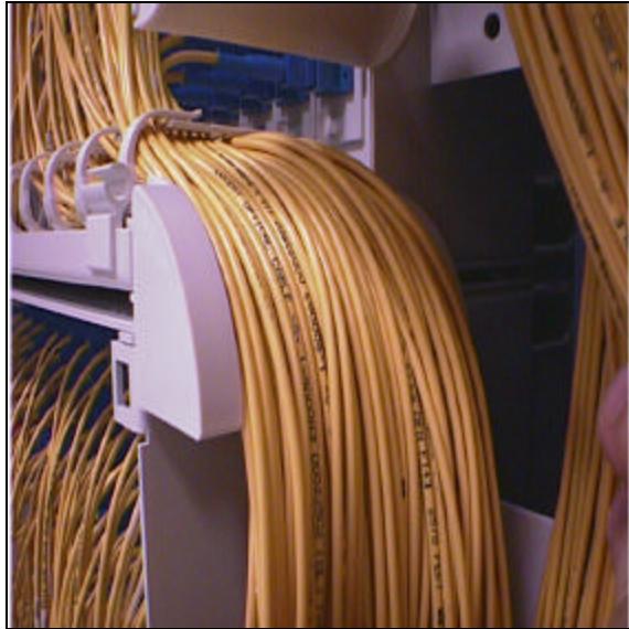
Fiber Distribution Shelf with SC 3.0-mm jumper.
